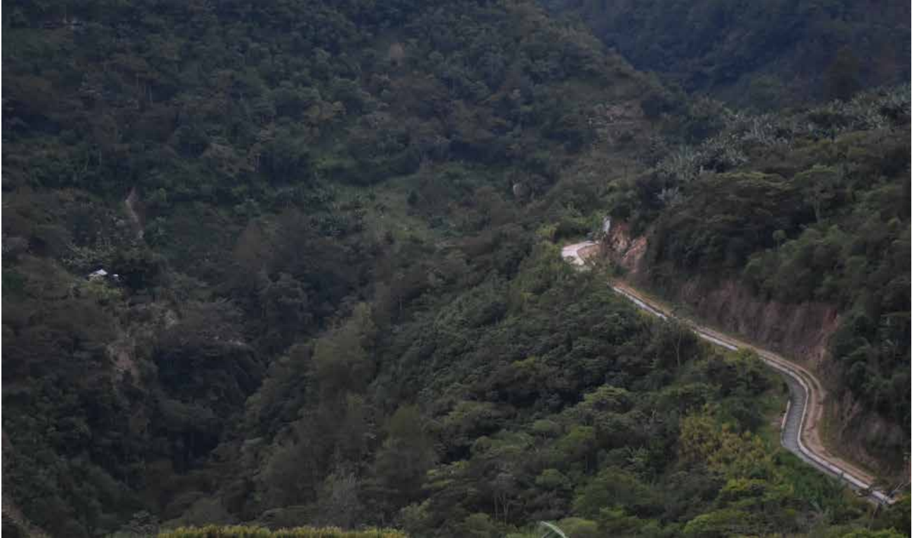
Canal of Aurora I hydroelectric dam. Water was granted in concession to Inversiones La Aurora S.A. de C.V company for 30 years.
