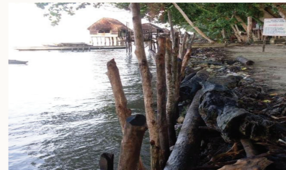
Figure 5. An example of a seawall built with local materials to prevent erosion (photo: Peter Bosip, July 2011)
