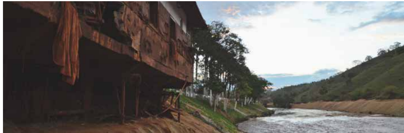
A year after the collapse of the dam, houses from different communities still show signs of the crime. A large house on the Rio do Carmo, part of Rio Doce, in Barra Longa municipality, Minas Gerais, November 2016.
