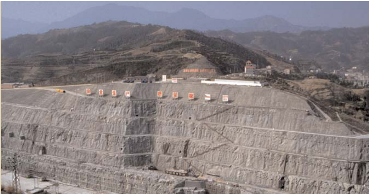
Three Gorges Dam, China.
