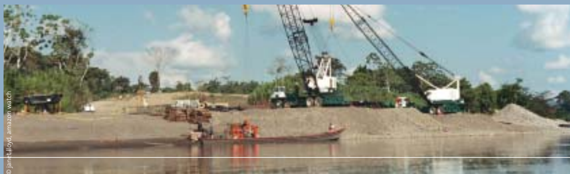
Cranes digging vast quantities of construction materials from the Unubamba river bank along the right of way for the Camisea gas pipeline in Peru, August, 2002
