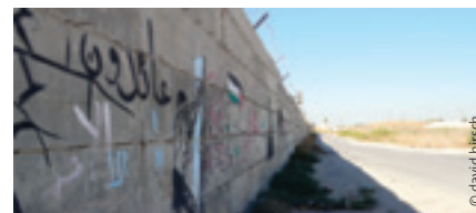
A part of the separation wall.
