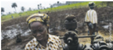
Oil Installation (The Christmas Tree). Ikot Ada Udo, Nigeria.
